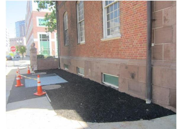
A bioretention system can be installed in front of the post office to capture, treat, and infiltrate rooftop runoff by redirecting the nearby downspout into it. A preliminary soil assessment suggests that more soil testing would be required before determining the soil's suitability for green infrastructure.
