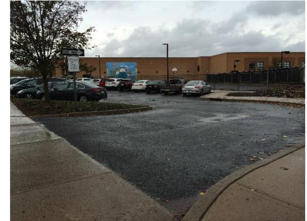
The building has internal drainage. Parking spaces can be replaced with porous asphalt to allow stormwater to infiltrate. A preliminary soil assessment suggests that more soil testing would be required before determining the soil's suitability for green infrastructure.
